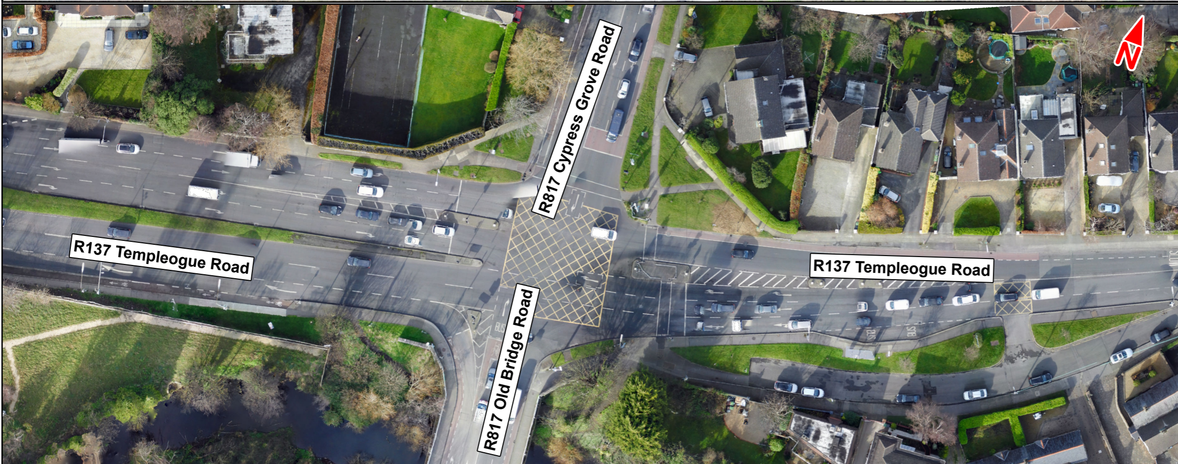
B) R137 TEMPLEOGUE ROAD / R817 CYPRESS GROVE ROAD AND OLD BRIDGE ROAD FOUR ARM SIGNALISED JUNCTION
